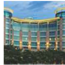
SHALIMAR TCS BUILDING
